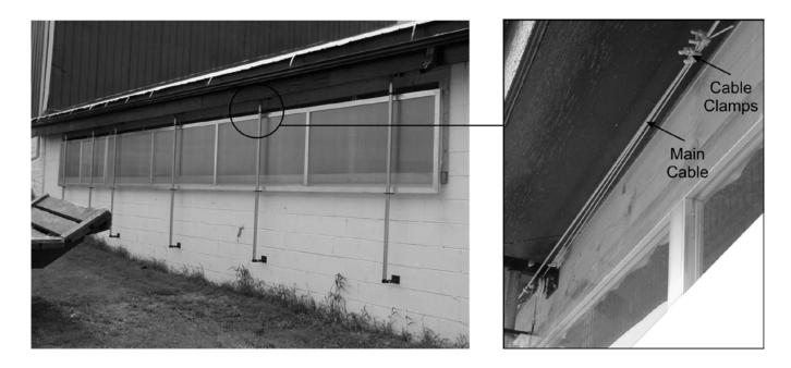
Double back secondary cable and standard secondary cable are clamped together to the main cable.
