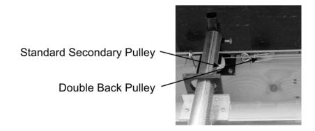
Secondary pull cable requiring a double back to allow travel into the end pulley and into the building.
