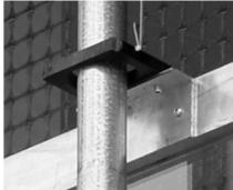
**11.** Operate the panel up and down to check for adjustments and that the secondary cables are plumb with the tracks. The clips used in the upper frame can be moved within the frame enabling this adjustment. You must then fasten the secondary track clip to the main panel frame using a self-tapping screw as shown.
